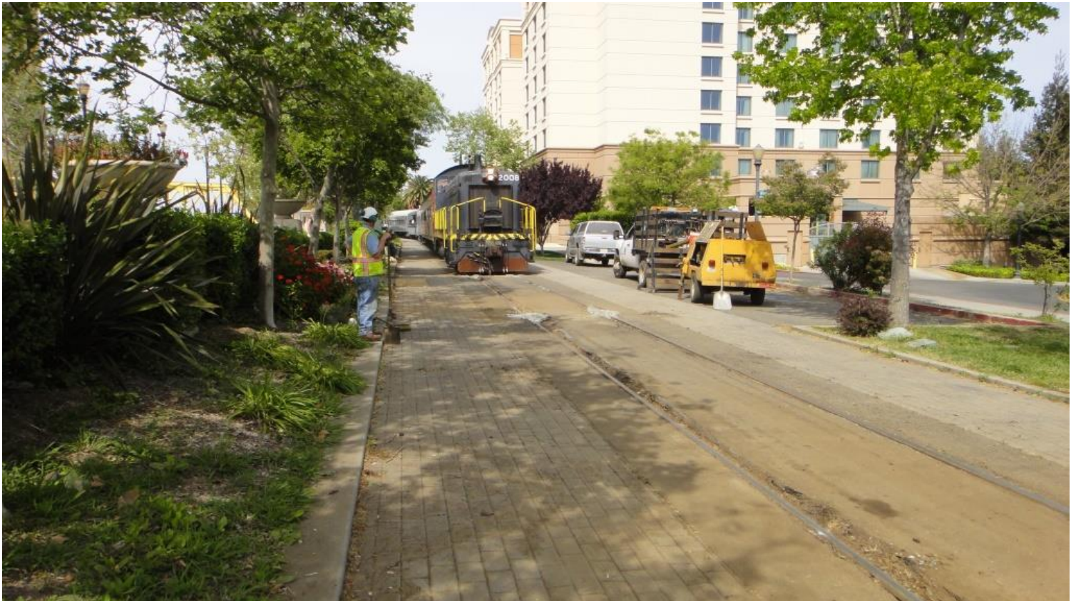
Crunch! As the 2008 rolled over the newly filled joint, lots of crunching sounds were heard as it crushed loose gravel in the flange ways
