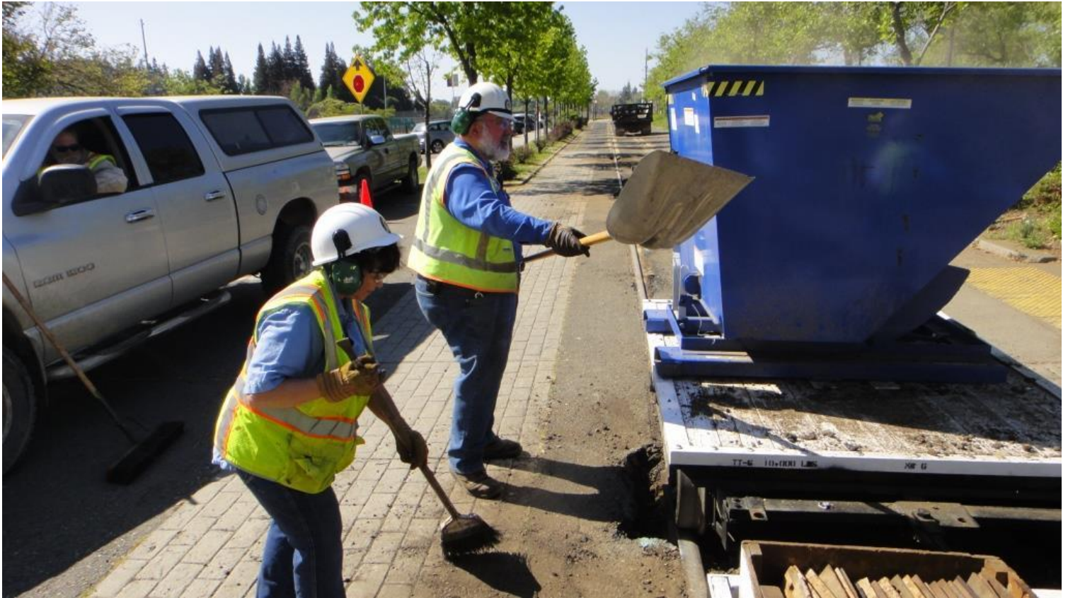
Pam and Frank transfer the debris from the ground into the dumpster
