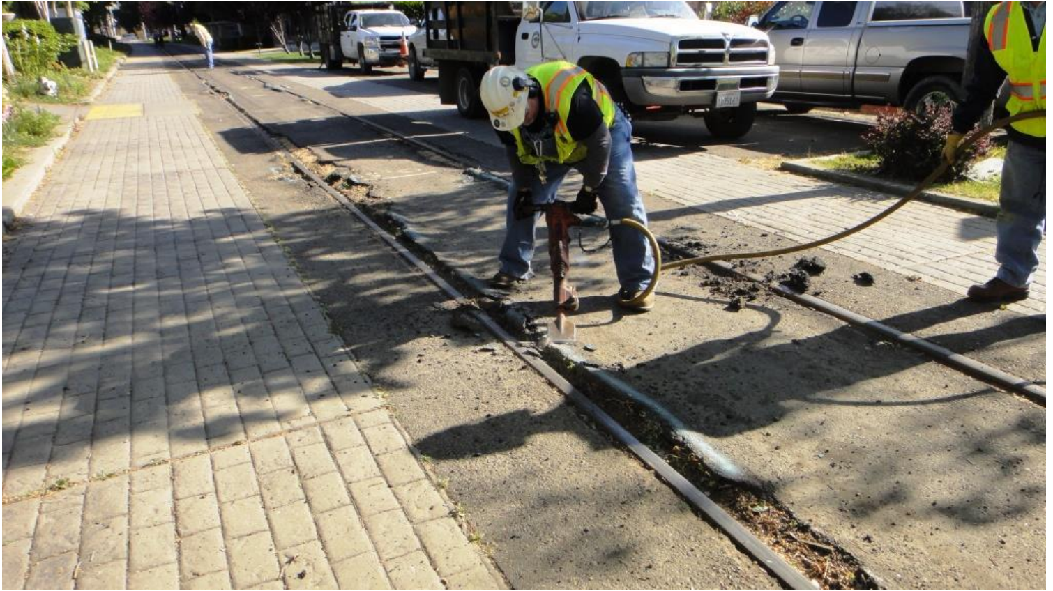
Mike F. using the spade-bit on the jackhammer shaves-off rippling asphalt along the flangeway
