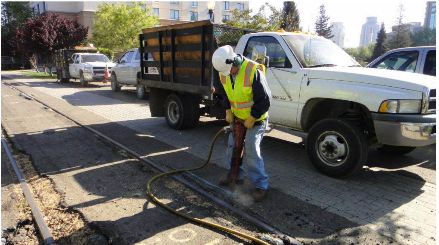
Mike W. cuts away at the asphalt around a rail joint
