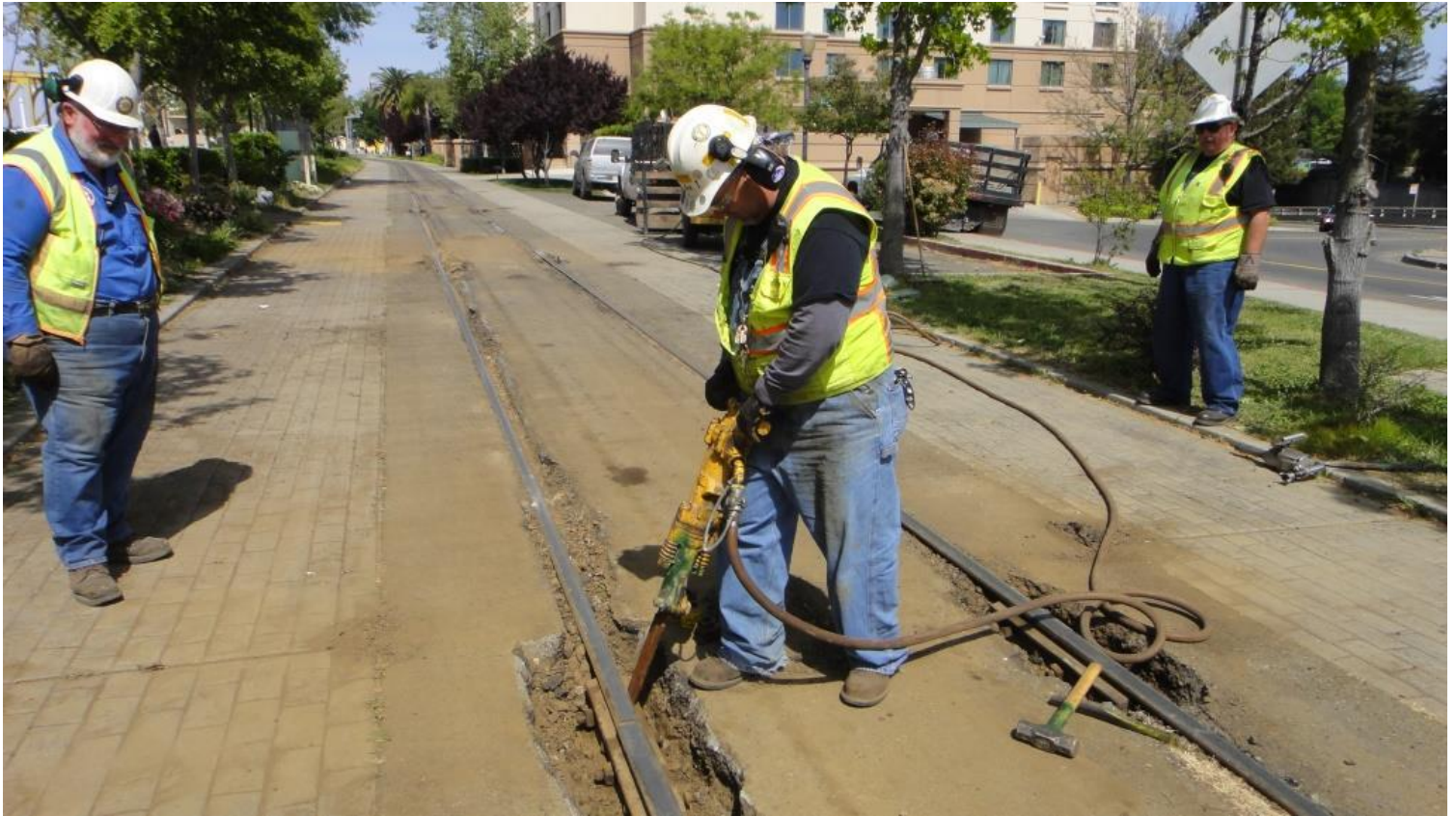
Mike F. taps the top of the joint-bar to shake out any debris caught between it and the web of the rail
