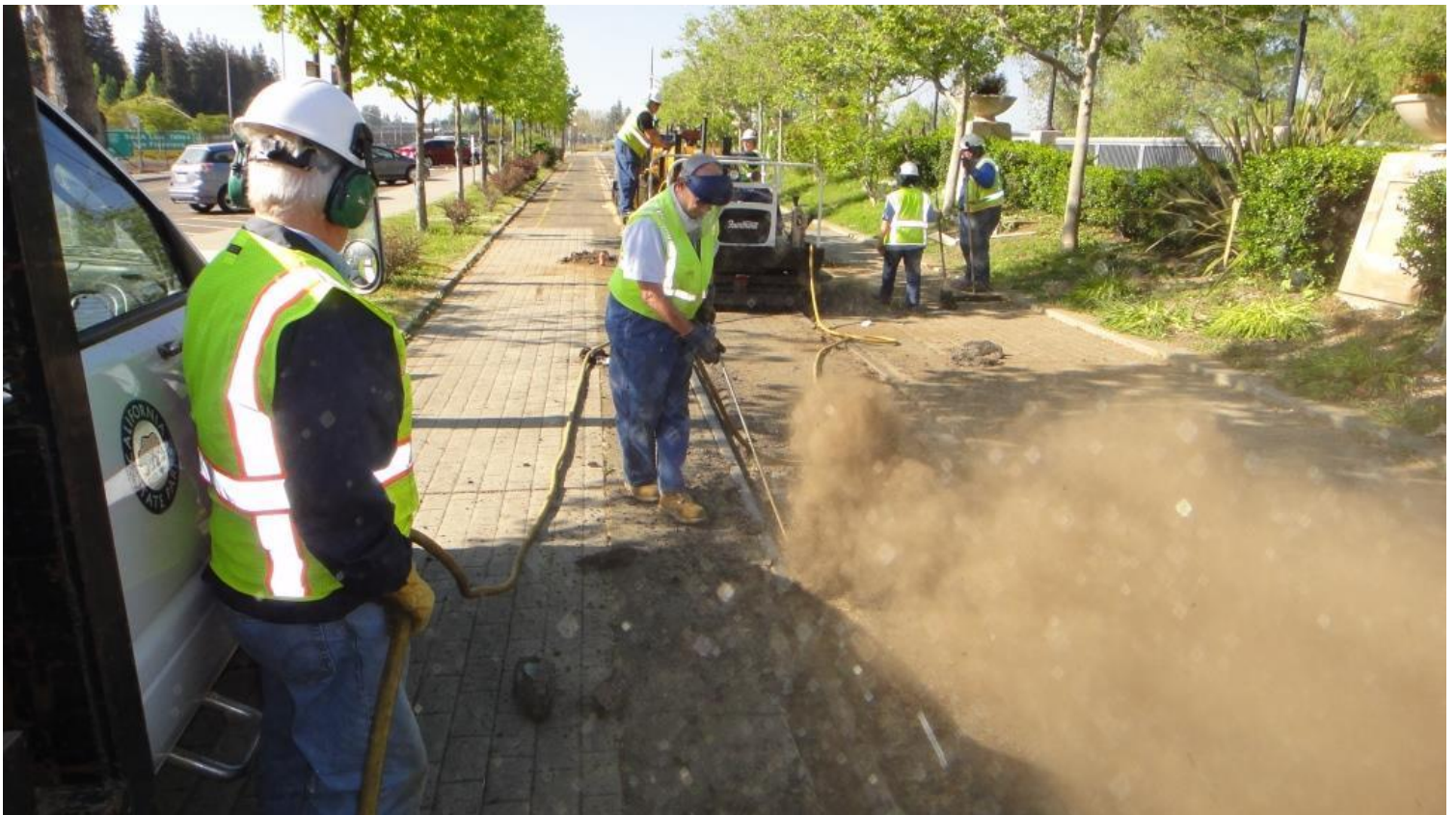
Clem blows all the crud and corruption out from around the rail-joint with the wand attachment on the air compressor
