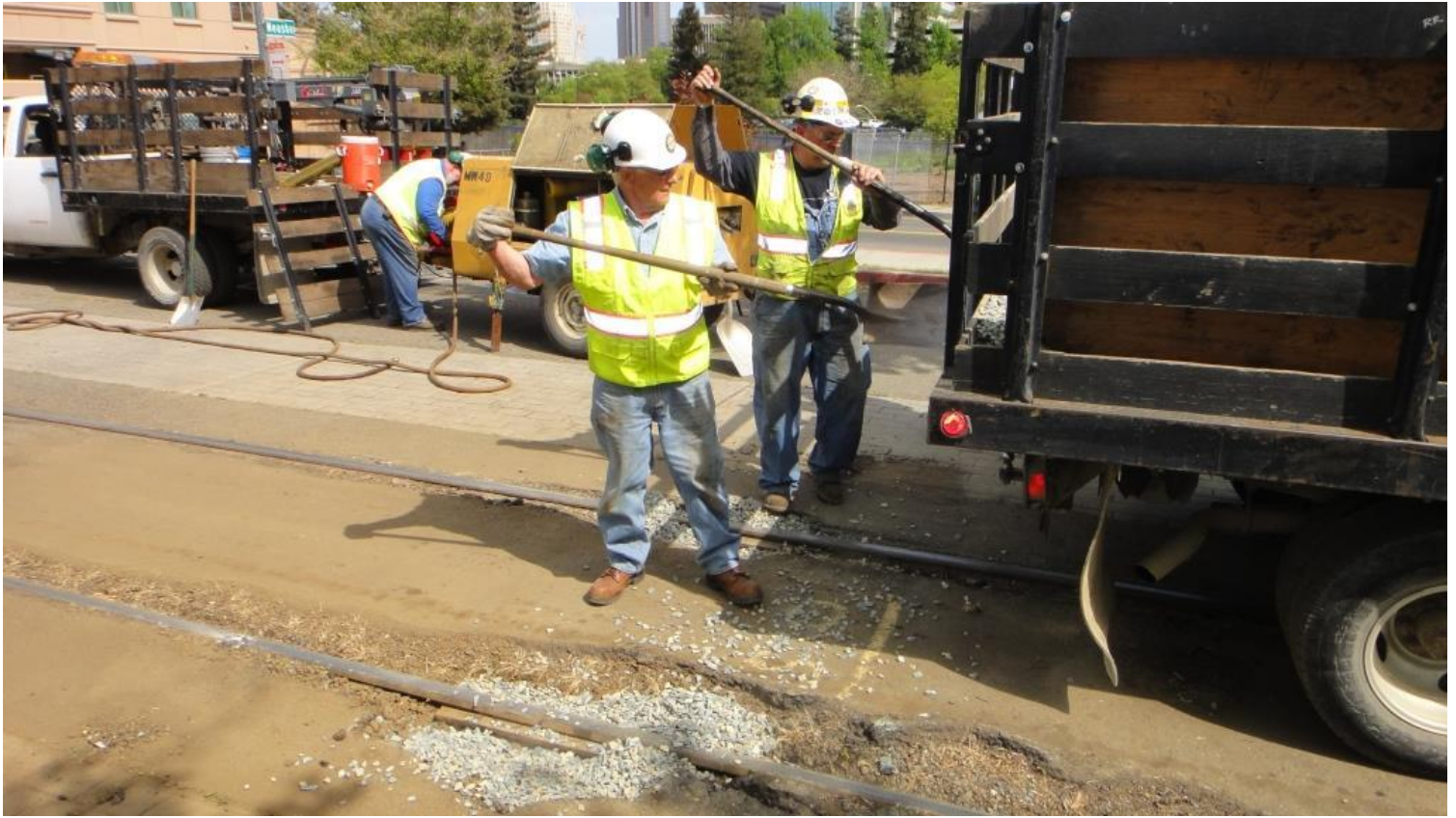
The two Mikes shovel pea-gravel into the holes around the exposed joints
